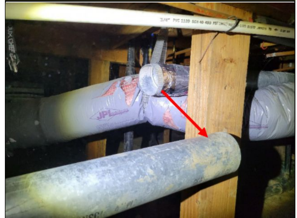
Item 38.1 - Clothes dryer duct disconnected.
