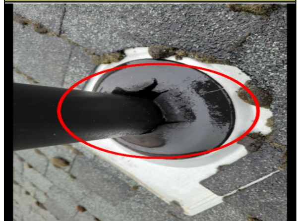
Item 1.4 - Split plumbing vent seal leaking
