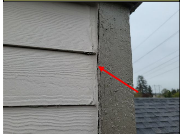
Item 8.1 - Split caulking on chimney chase, peeling paint.
