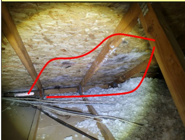
Item 1.5 - Mold and deterioration to OSB roof sheathing
