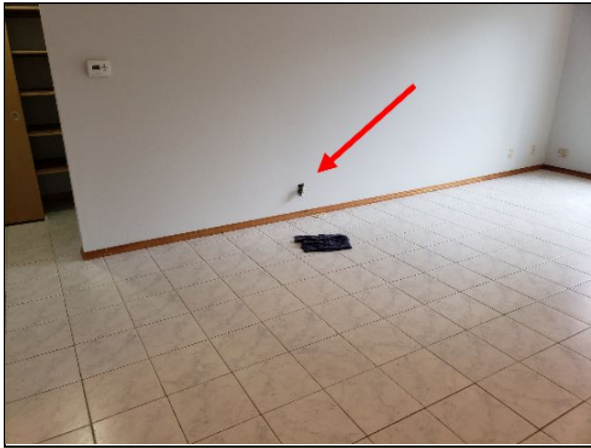
Item 9.2 - Receptacle hanging by wiring: One in family room.
