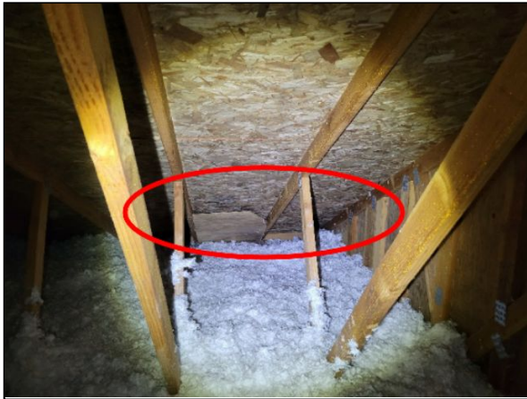
Item 1.13 - Mold and deterioration to OSB roof sheathing
