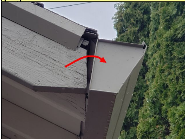
Item 34.1 - Loose gutter: Front right corner.
