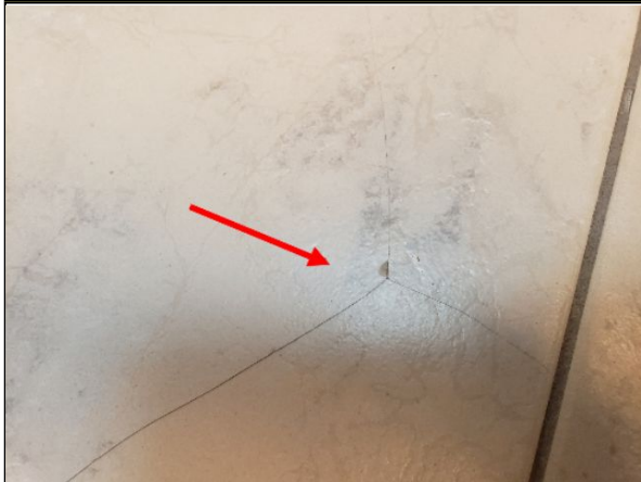
Item 28.6 - Cracked floor tiles: Master bedroom bathroom.
