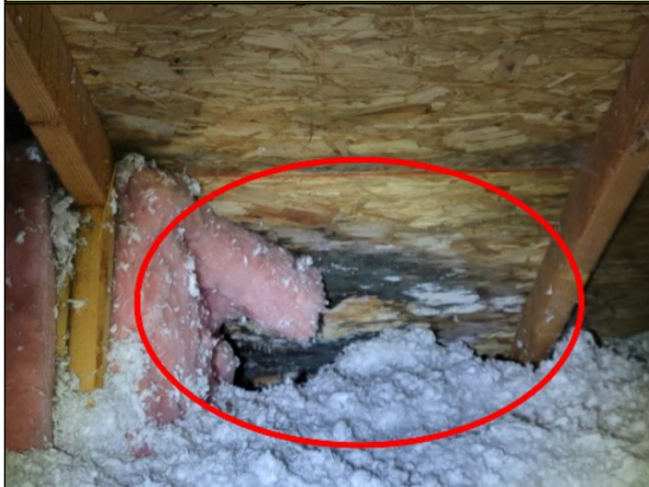
Item 1.11 - Mold and deterioration to OSB roof sheathing
