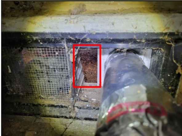
Item 39.1 - Gaps/openings in crawlspace vent around clothes dryer duct.
