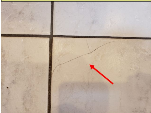
Item 28.2 - Cracked floor tiles: Kitchen.
