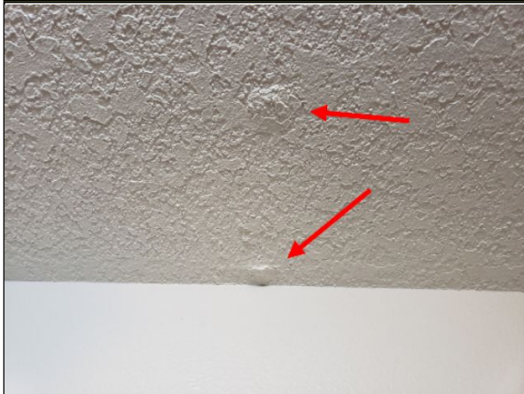
Item 32.1 - Drywall nail pops - ceilings: Hallway outside of hallway
