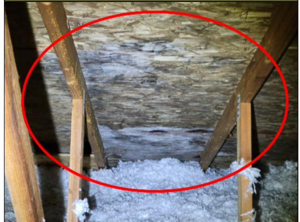
Item 1.12 - Mold and deterioration to OSB roof sheathing
