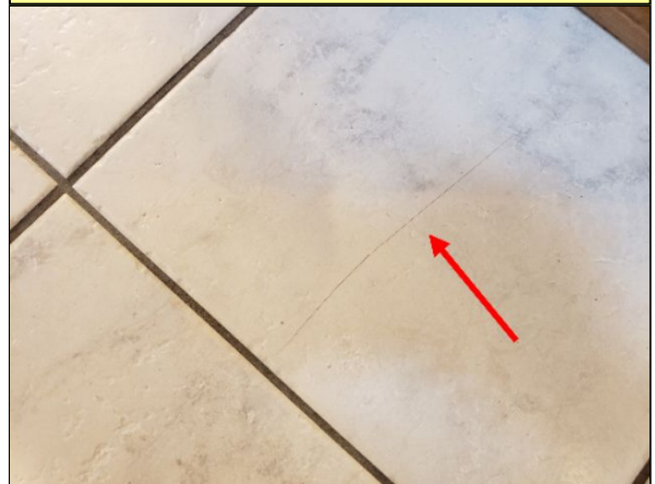
Item 28.3 - Cracked floor tiles: Kitchen.
