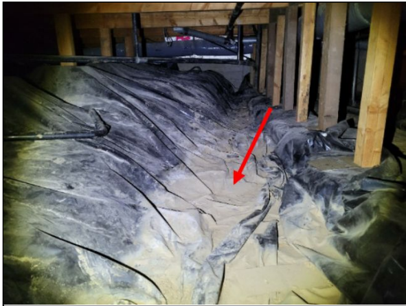
Item 23.2 - Silt on vapor barrier in crawlspace.
