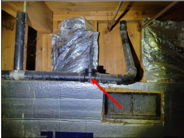
Item 4.1 - Cracked drainage fitting in crawlspace.
