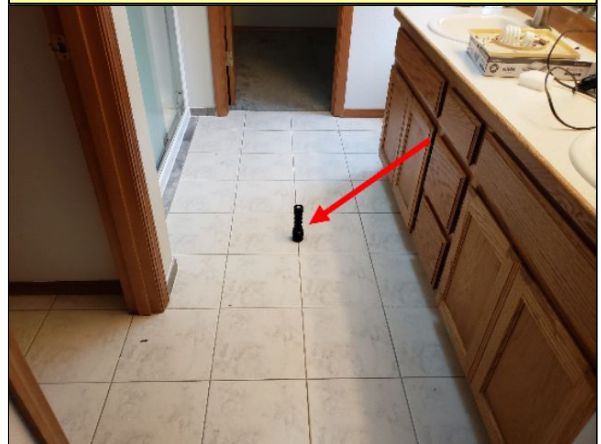
Item 29.2 - Popped grout floor tile joint: Master bedroom bathroom.
