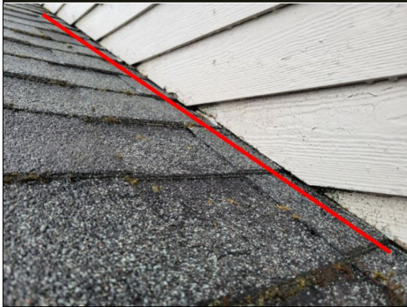
Item 7.3 - Siding and sheathing too close to roof: On back of home along
