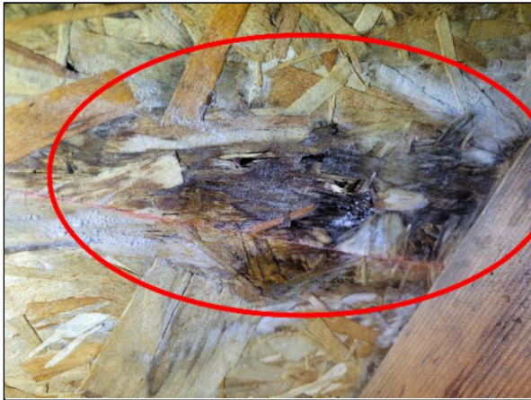
Item 1.7 - Mold and deterioration to OSB roof sheathing
