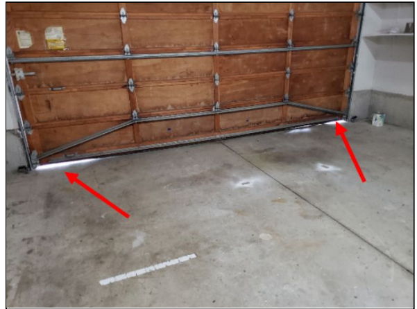
Item 26.1 - Daylight through garage door bottom seal.
