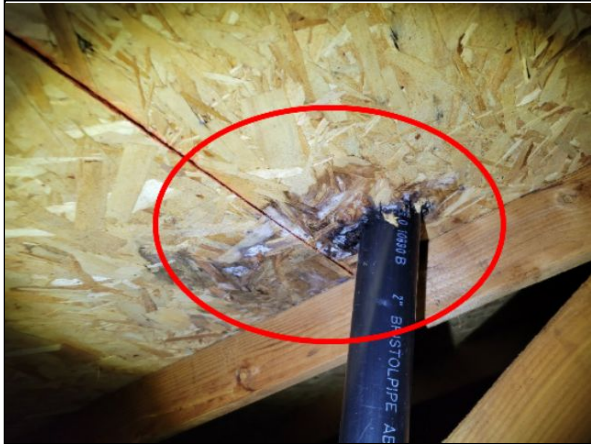
Item 1.9 - Old roof, leaks at some plumbing vents
