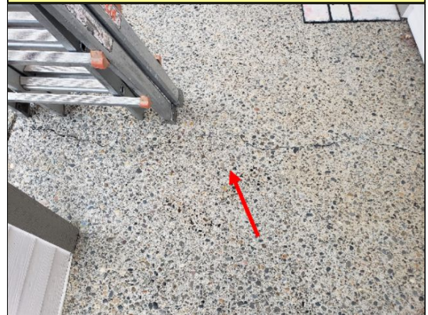
Item 40.1 - Cracked concrete front porch.
