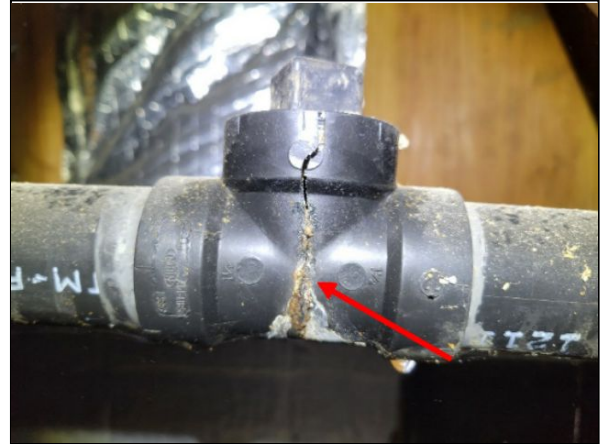
Item 4.2 - Cracked drainage fitting in crawlspace.
