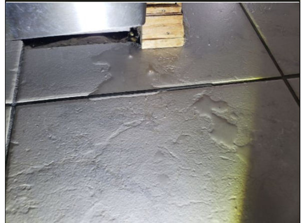
Item 33.1 - Dishwasher leaking at door.
