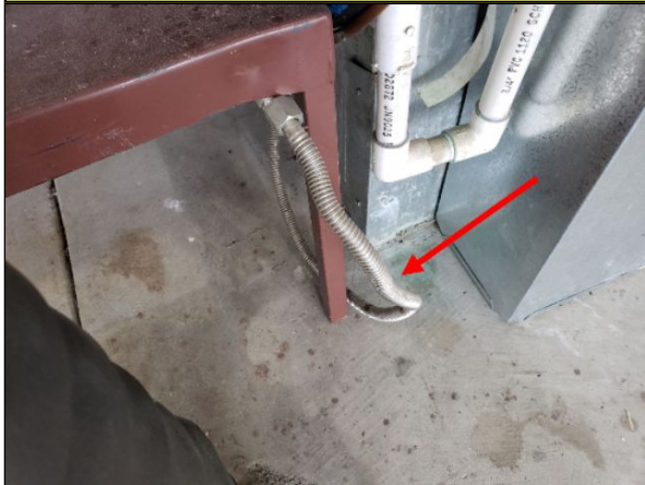
Item 51.1 - Abandoned gas line for a clothes dryer.
