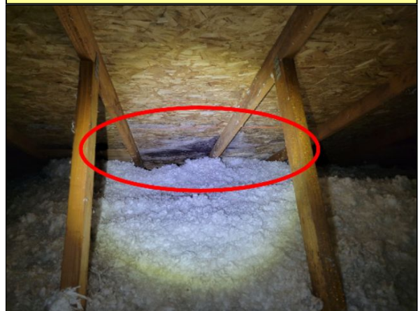
Item 1.6 - Mold and deterioration to OSB roof sheathing
