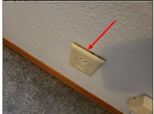
Item 15.1 - Loose receptacle: Under window in the 2nd bedroom.
