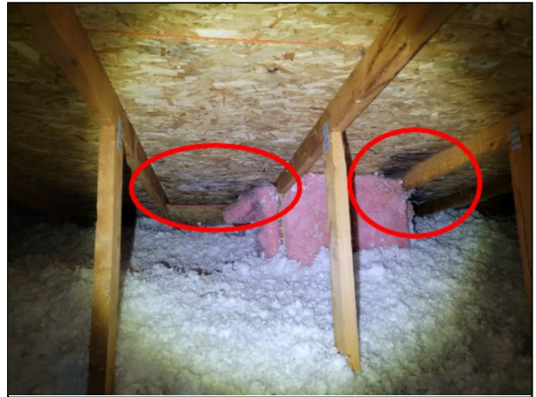
Item 1.8 - Mold and deterioration to OSB roof sheathing
