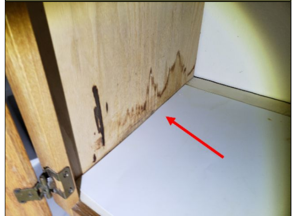
Item 48.1 - Moisture stains in cabinet: In hallway bathroom sink cabinet.
