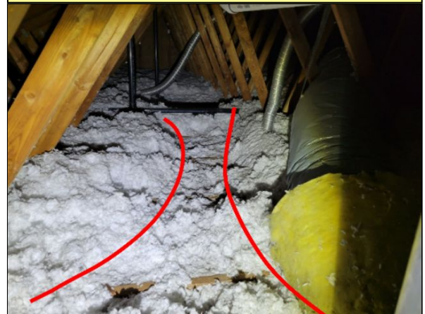
Item 35.1 - Disturbed insulation in the attic.
