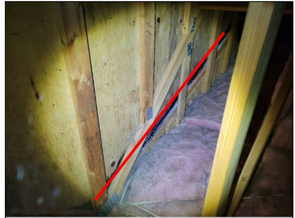
Item 7.2 - Rot/moisture damaged plywood wall sheathing.
