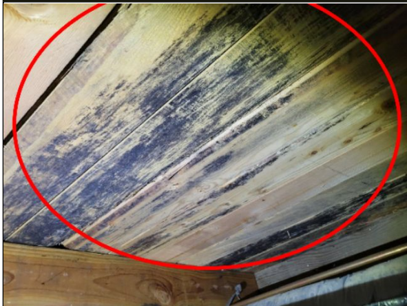
Item 24.1 - Lumber mold on beams in crawlspace.
