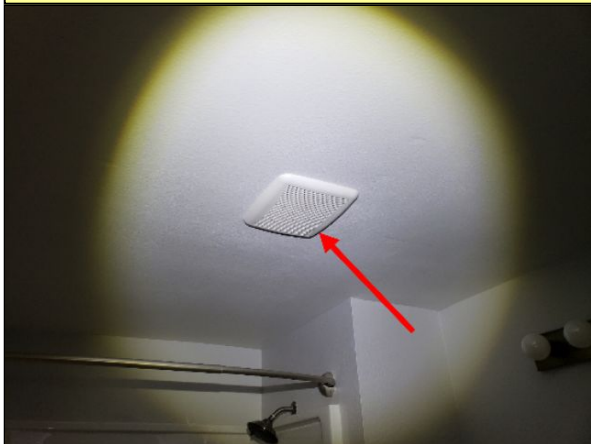
Item 12.1 - Bathroom exhaust fan not working: Hallway bathroom.
