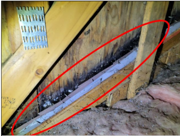
Item 7.1 - Rot/moisture damaged plywood wall sheathing.
