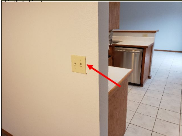
Item 14.3 - Mis-wired two way lighting circuit: For kitchen ceiling
