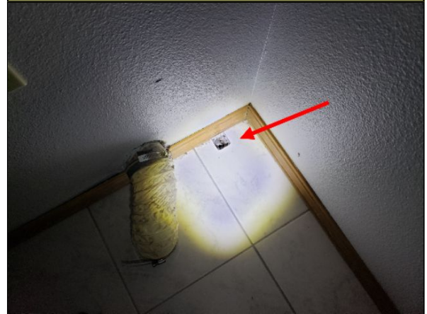
Item 51.2 - Abandoned gas line for a clothes dryer.
