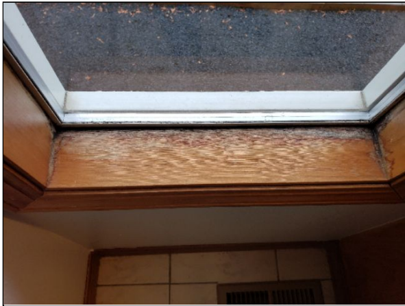
Item 49.1 - Moisture stains on window sill.
