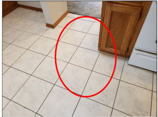
Item 28.5 - Cracked floor tiles: Kitchen.
