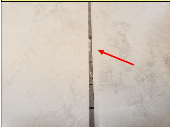
Item 29.1 - Popped grout floor tile joint: Master bedroom bathroom.
