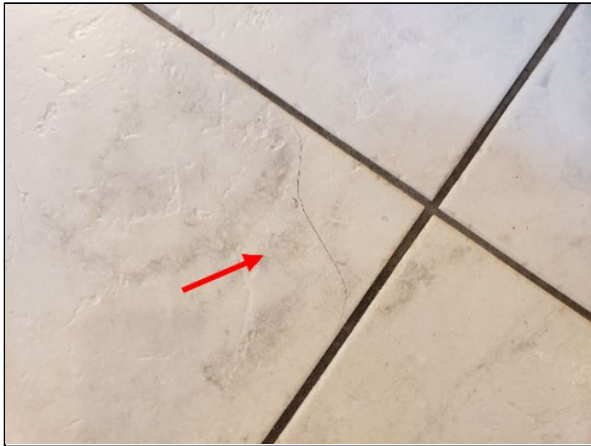
Item 28.4 - Cracked floor tiles: Kitchen.
