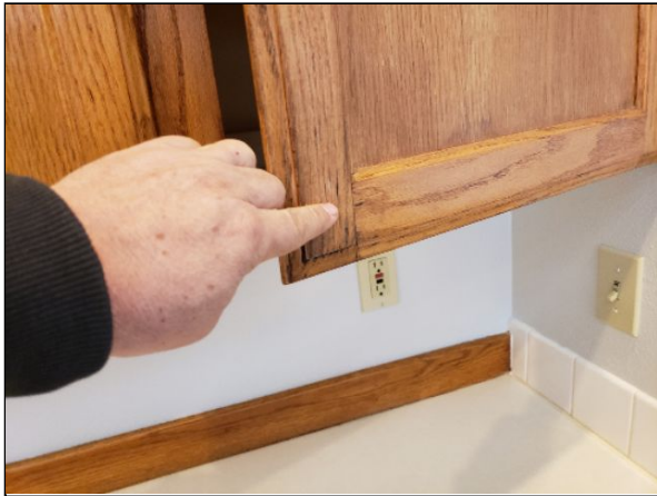
Item 36.1 - Joint separation in cabinet door.
