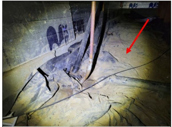
Item 23.3 - Silt on vapor barrier in crawlspace.
