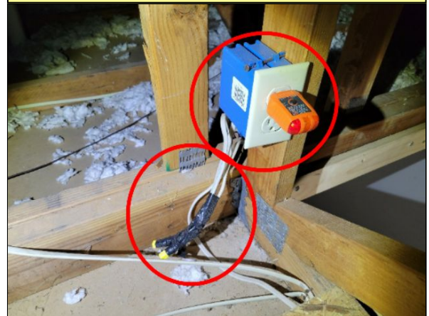
Item 13.1 - Improperly wired in receptacle: In attic over the garage.
