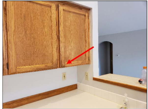
Item 36.2 - Joint separation in cabinet door.
