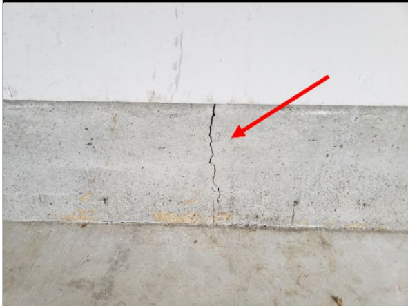
Item 44.1 - Common shrinkage cracks in foundation.
