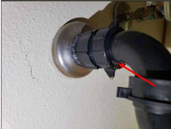
Item 5.1 - Trap arm to branch drain connection leaks: 1st sink in master bedroom bathroom.
