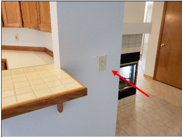
Item 14.1 - Mis-wired two way lighting circuit: For kitchen ceiling
