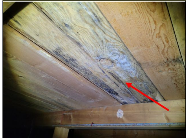
Item 24.2 - Lumber mold on subflooring in crawlspace.
