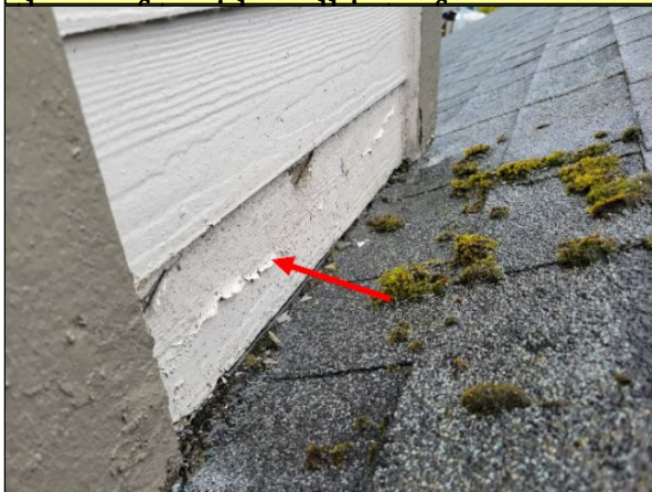
Item 8.2 - Split caulking on chimney chase, peeling paint.
