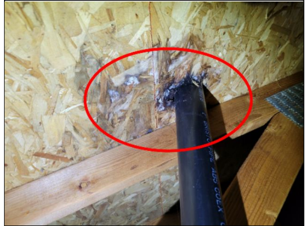
Item 1.10 - Old roof, leaks at some plumbing vents
