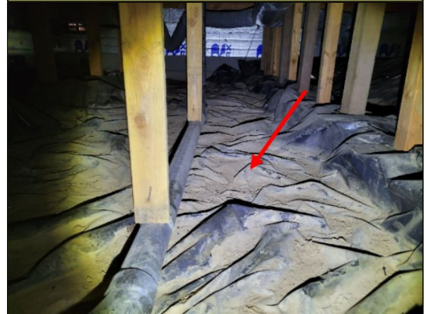
Item 23.1 - Silt on vapor barrier in crawlspace.
