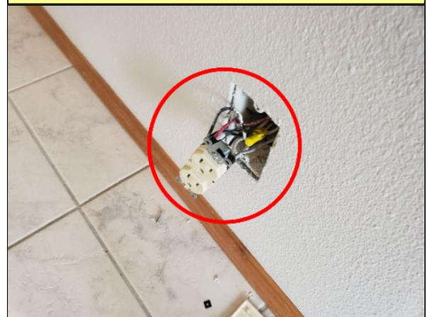
Item 9.1 - Receptacle hanging by wiring: One in family room.
